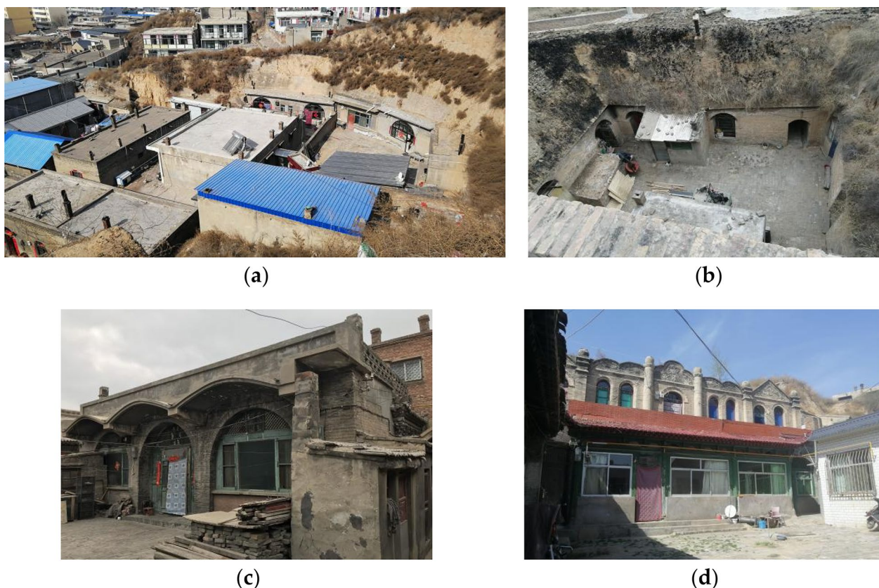
Fig. 5 Cave-dwellings in Puhuiquan Neighborhood: a Wraparound cliff cave-dwelling; b Underground cave-dwelling courtyard; c Independent cave-dwelling; d Special independent cave-dwelling with the cave arch downstairs and the Chinese classical beam-column structure upstairs
